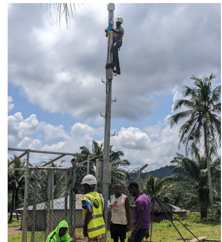
Construction on a new cell tower in Big Jay, Liberia | 2022
